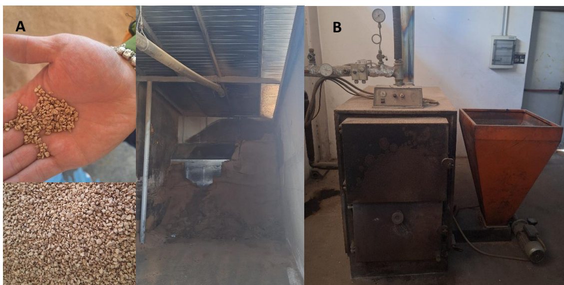
Fig. 2. The olive stones produced by the cooperative (A) and the water heater used to produce hot water onsite(B)
